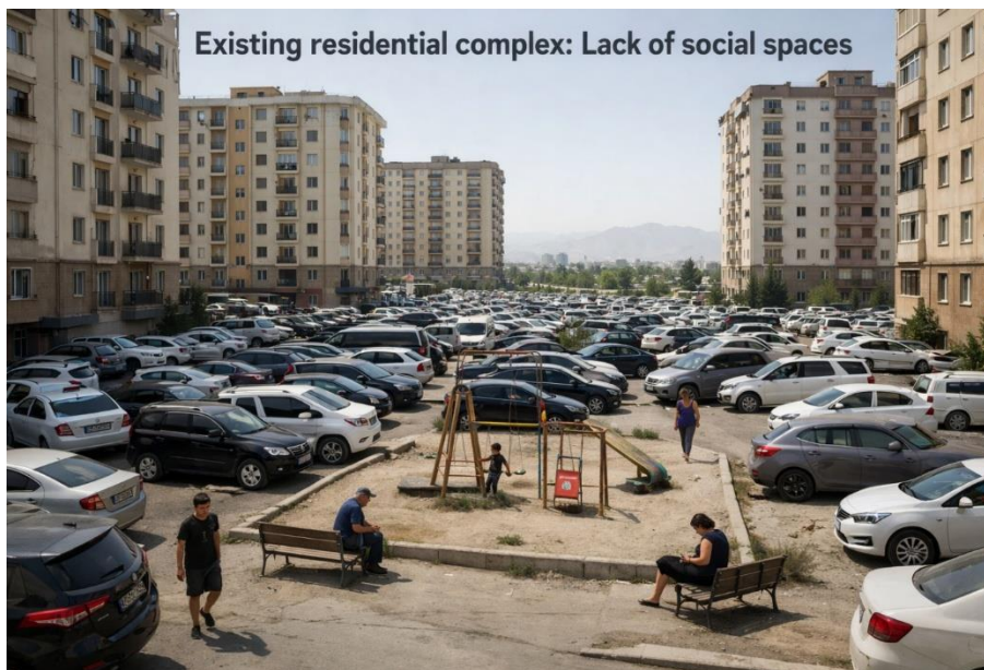
Figure 3. DARBON/DURMON EXISTING CONDITIONS
